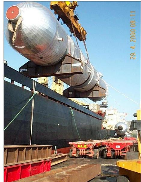
Discharge from ship to SPMT's on a barge
